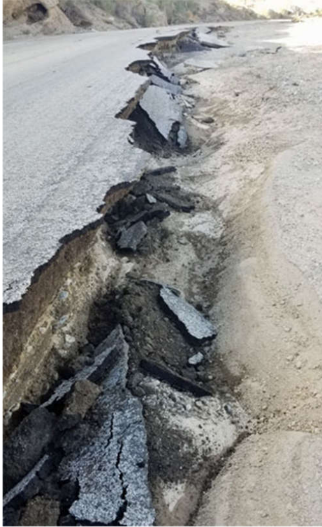
Road Undermined Photo by Eric Holden.
